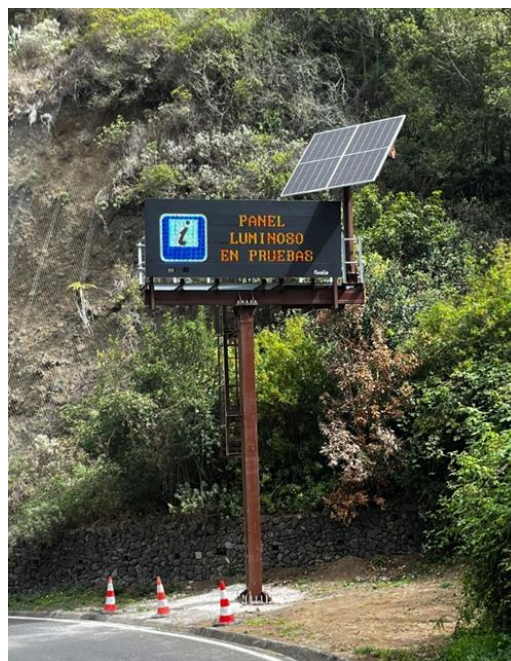
Figure 3. Autonomous VMS with embedded LPR camera (La Gomera, Canary Islands, Spain)
